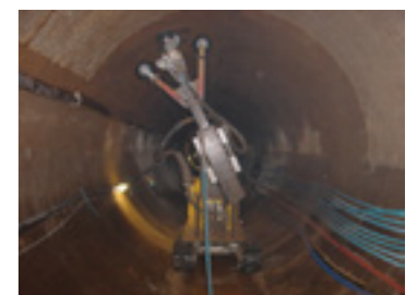
The Robot in sewage tunnel. Paris, France
