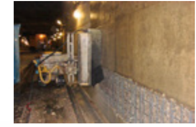
Robot removing concrete from a tunnel wall. Stockholm, Sweden.
