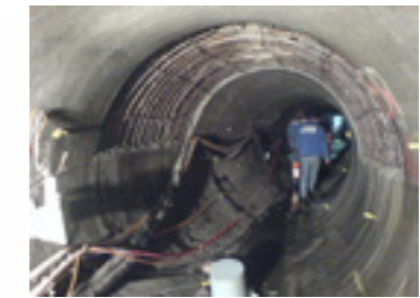
Result of hydrodemolition with Robot in a tunnel. Zürich, Switzerland
