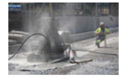
Robot removing concrete from a bridge deck. Stockholm, Sweden.
